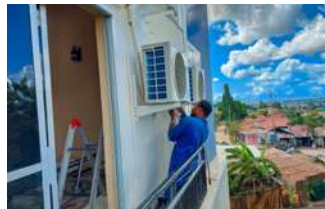
Installing an outdoor unit on a house
