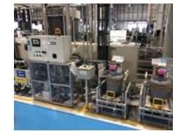
Recovering refrigerant in the production process
